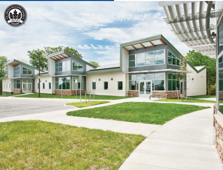
▲ Loudoun County Youth Shelter features geothermal wells and extensive photovoltaic panel arrays.
