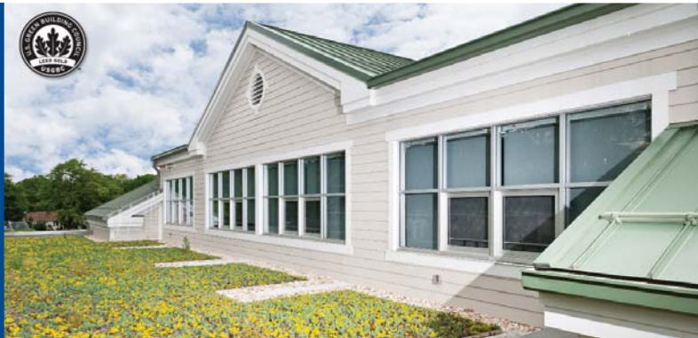
▼ Great Falls Fire Station #12 features a vegetative roof and in-slab radiant heating.
